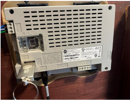
FIG. 1 - USB CONNECTION TO HMI
